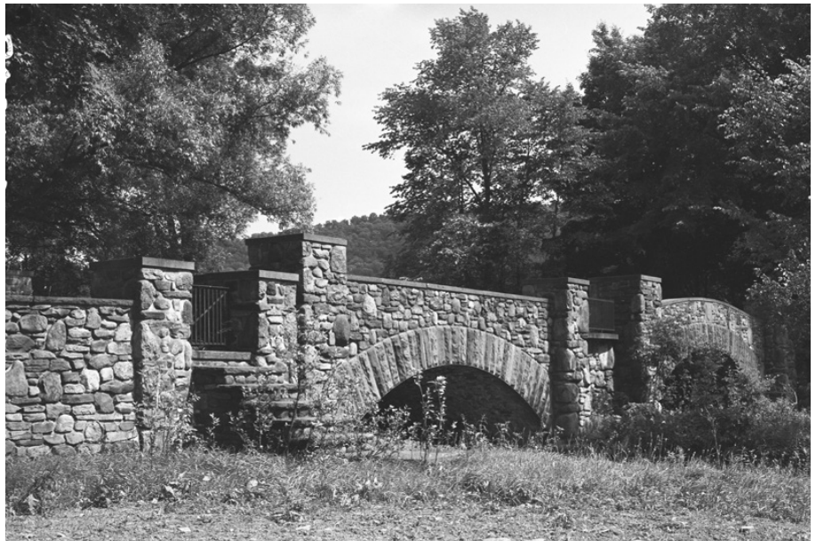
McLean Bridge in South Kortright Bridge, July 1947; Bob Wyer photo contributed by DCHA.
